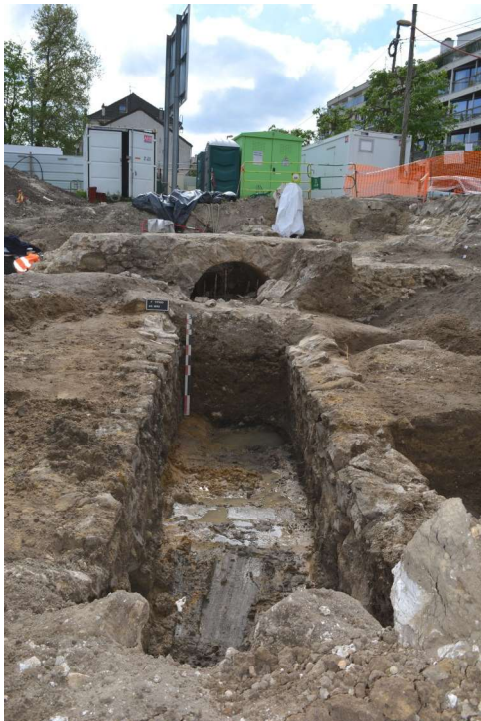
Fig.8 Egout maçonné du XIX e siècle, C. Seng (Inrap)
